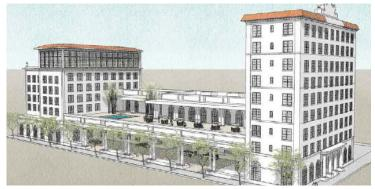
This broader rendering above shows how the existing Terrace Hotel (at top right) is connected to the proposed residential tower (at top left) by the amenity deck. The lower level of the deck is lobby, drop-off, and garage level access.
